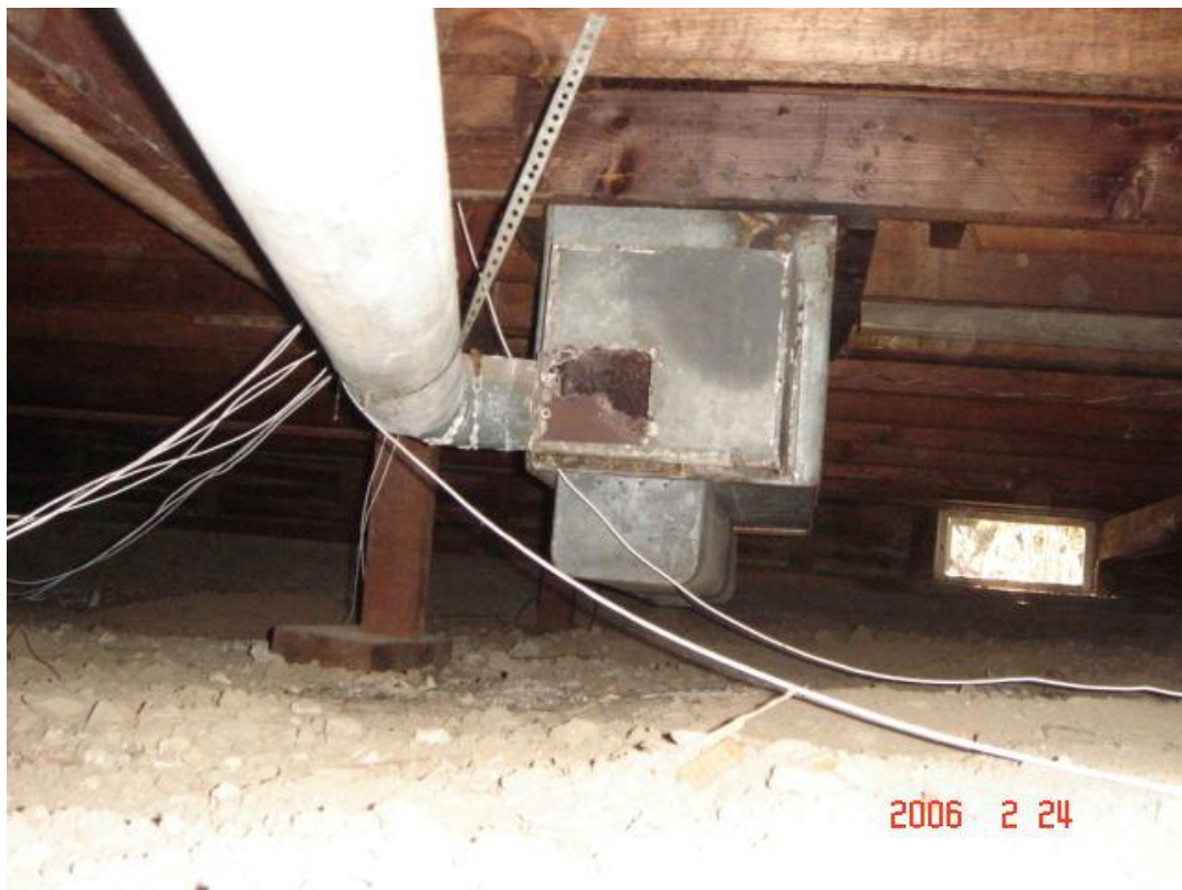
Improper drain fitting under the hall bathroom.
