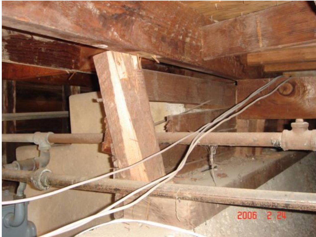
Loose cripple wall support.
