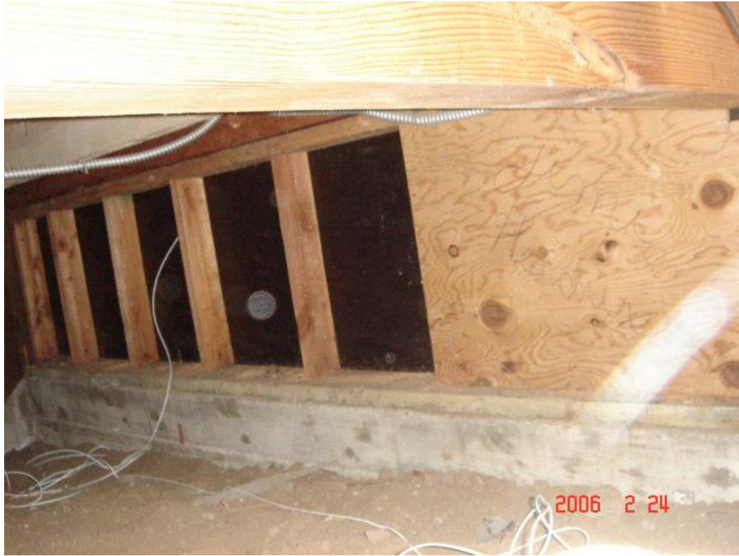
Partial incorrectly installed shear wall support.
