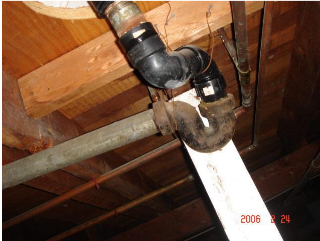
Improper drain fitting under the hall bathroom.
