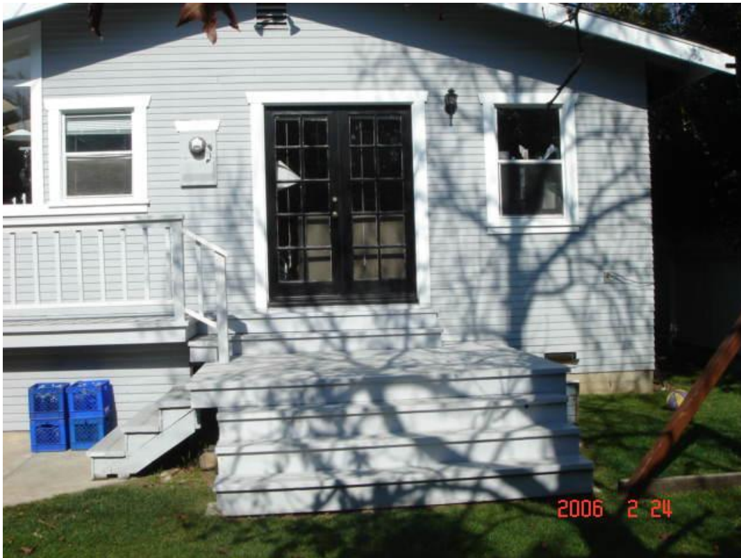
The rear view of the house. The deck is under 30 inches, no guardrail required.
