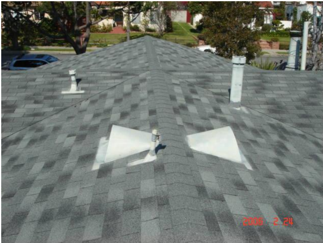
The roof in good condition.
